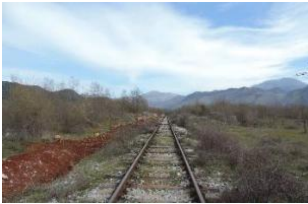
Figura 45: Km 132+620 to km 133+370
